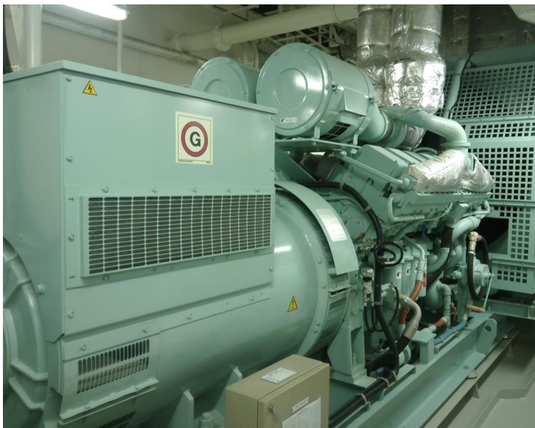
Slika 15 Emergency generator
