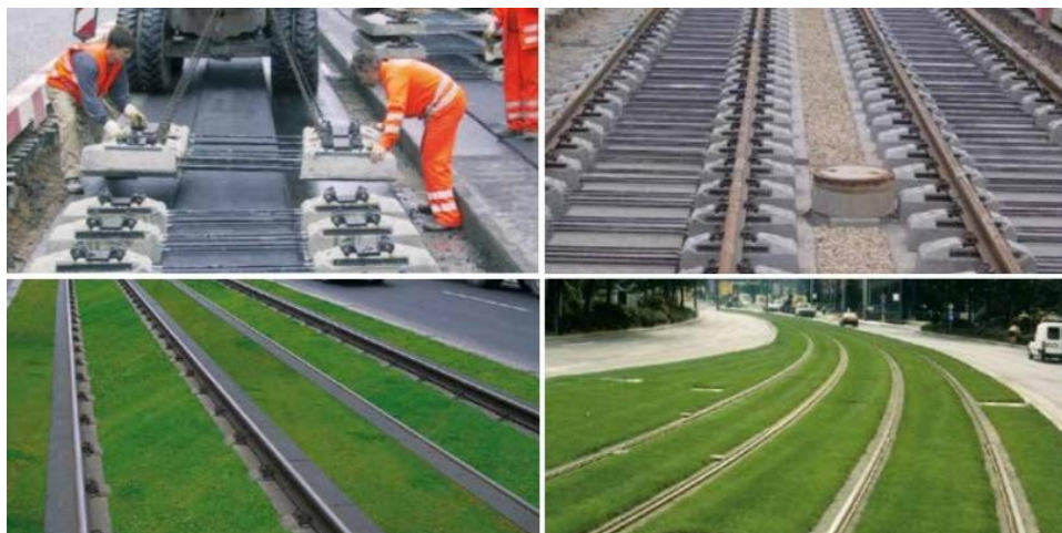
Slika 6. Sistem „ATD–G“ sa zelenim pokrivačem u Berlinu ( https://www.railone.com/fileadmin/daten/05-presse-medien/downloads/broschueren/en/Green_tracks_EN_2011_ebook.pdf , 20.08.2021.)
