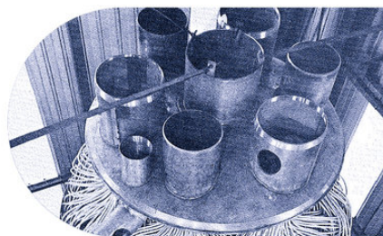
Air Liquide Coil Wound technology was used on Skidda plant in 1964
