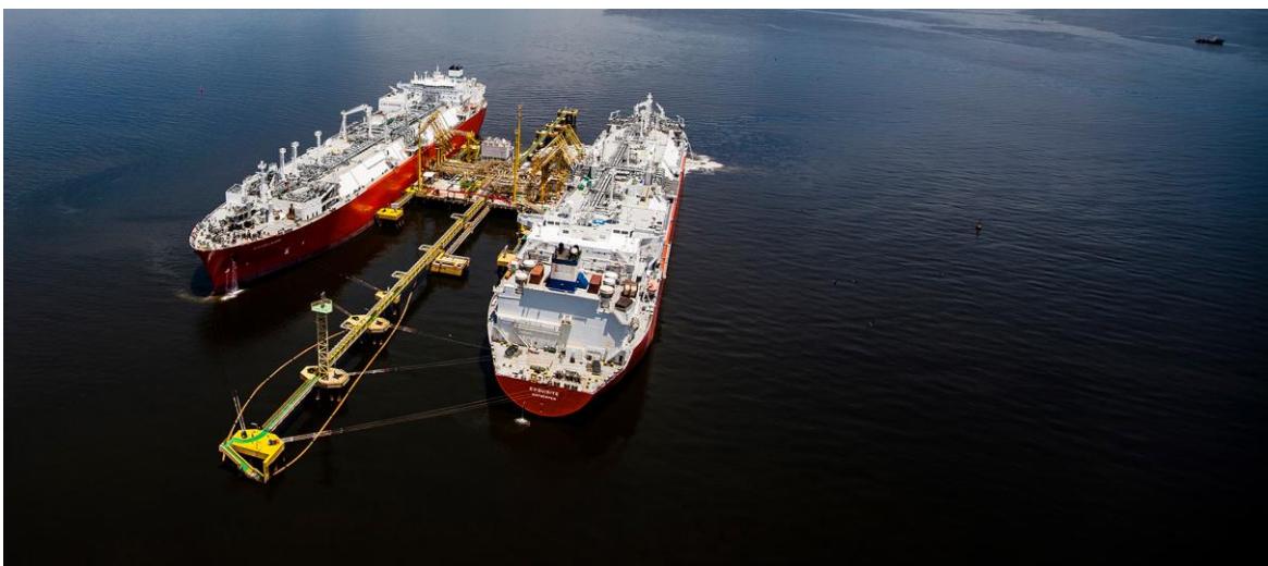
Slika 5: Cross jetty mooring
