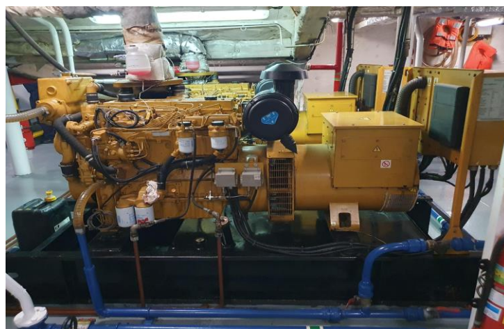
Slika 10. Caterpillar Olympian dizel generator
