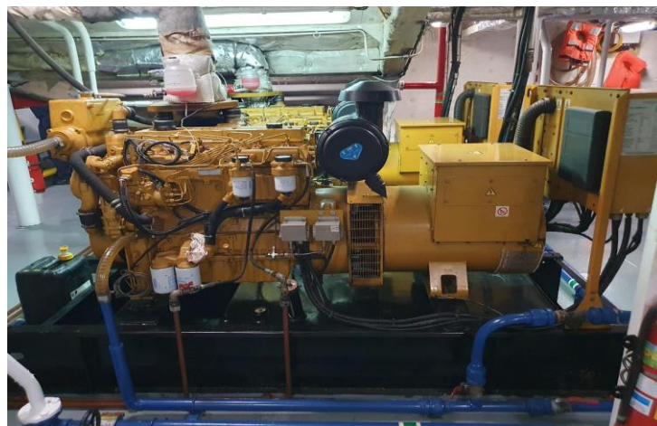
Slika 10. Caterpillar Olympian dizel generator
