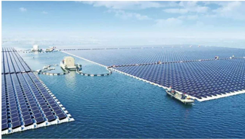
Figure 5. Floating solar plant. [5]
