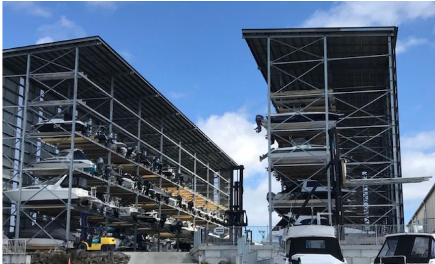
Slika 17 Regalno skladište Tamaki marine parka u Aucklandu, Novi Zeland Izvor: https://www.tamakimarinepark.co.nz/drystack/
